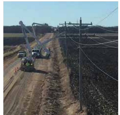
Prairie Energy crews worked in the Duncombe Substation area to replace bad insulators, add lightning arrestors, and place armor rod to the conductors. These improvements will help guard against bending, abrasion, arcing, and compression.
